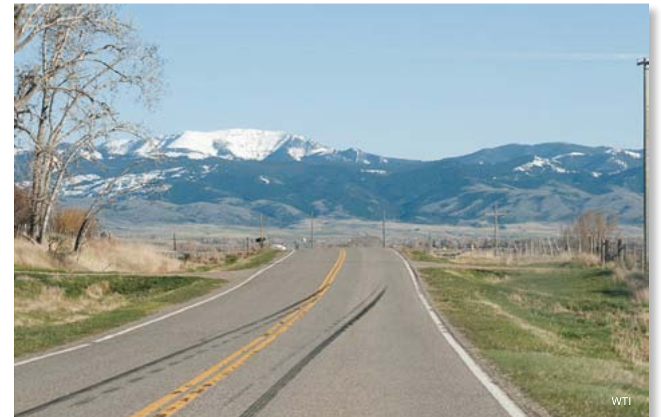
Visual indications, such as skid marks, can identify potential safety issues during a field audit.
