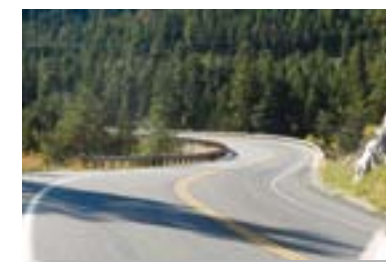
Figure 1: Horizontal Curve Guardrail. Photo by William Shorb.
