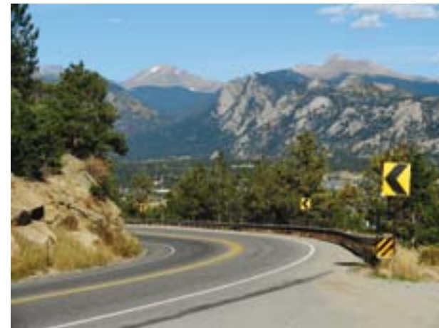
Chevrons improve curve delineation and provide warning of an alignment change. Photo by William Shorb.
