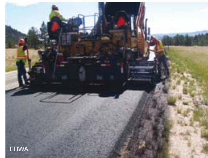
Installation of the Safety Edge SM coincides with the paving operation.
