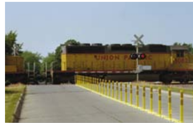
Figure 2: Railroad-highway crossing with lane separators. Photo by Peter Speer.
