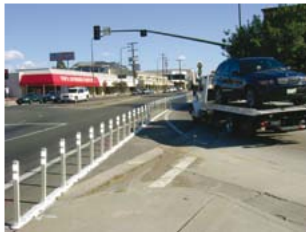
Figure 1: Lane separators for through and right-turn lanes. Photo by Peter Speer.
