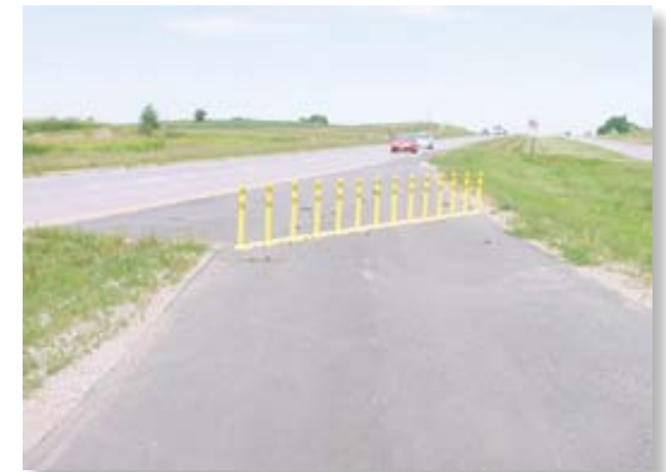
Figure 3: Median closures using lane separators. Photo by Peter Speer.
