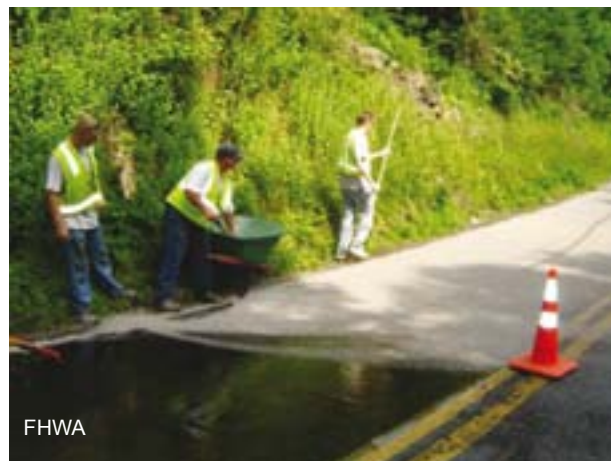
Installation of high friction surfaces manually and mechanically.
