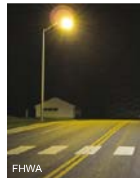
Lighting provides the driver with a visual indication of the presence of an intersection.
