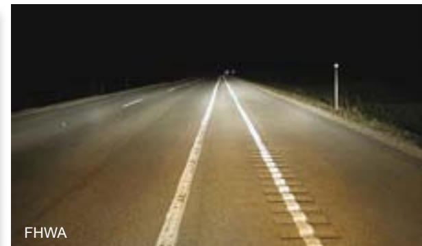
Rumble strips and stripes provide warning that a vehicle has left the travel lane. Rumble stripes also aid in enhancing edgeline visibility.
